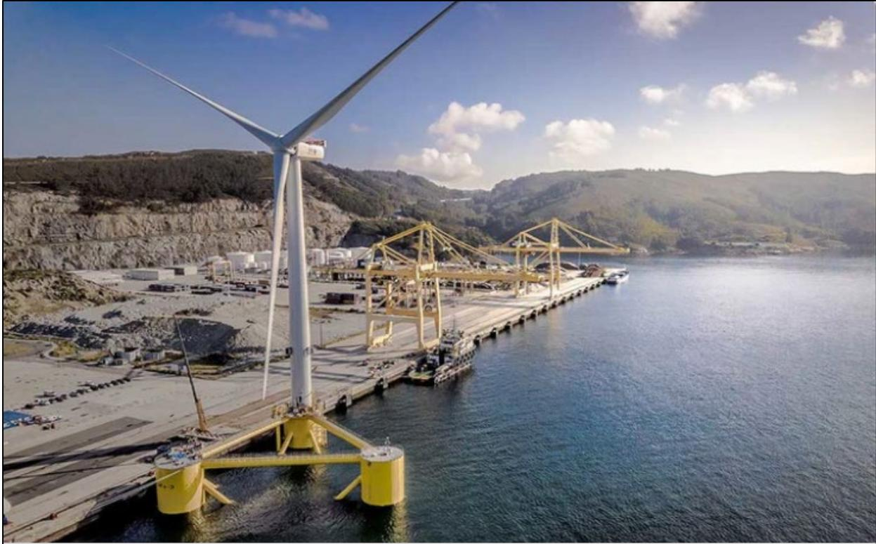
**Figure 3: WTG components assembled on semi-submersible foundation at quayside. Source: Principle Power**
