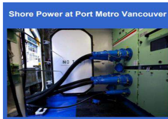
Figure 4: Shore power services at Port of Metro Vancouver (The Port of Metro Vancouver, 2017)
