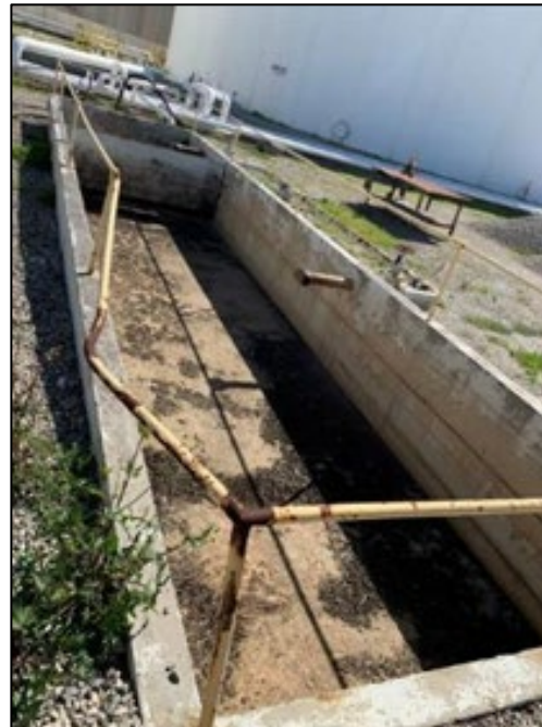
Figure 1-6. Concrete Oil/Water Separator Sump (to be demolished)
